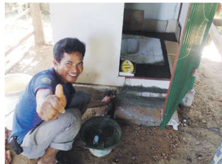
Top left: The DIY toilet being built. Top right and above: The finished product.
